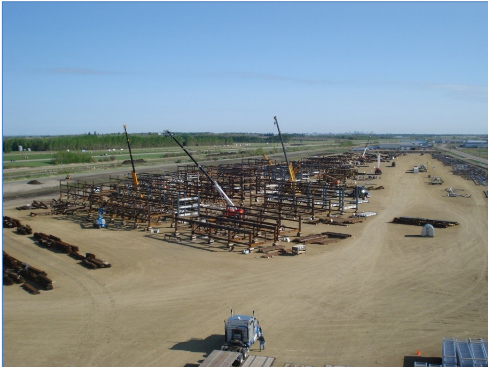
Figure 2-1 A typical module yard layout
