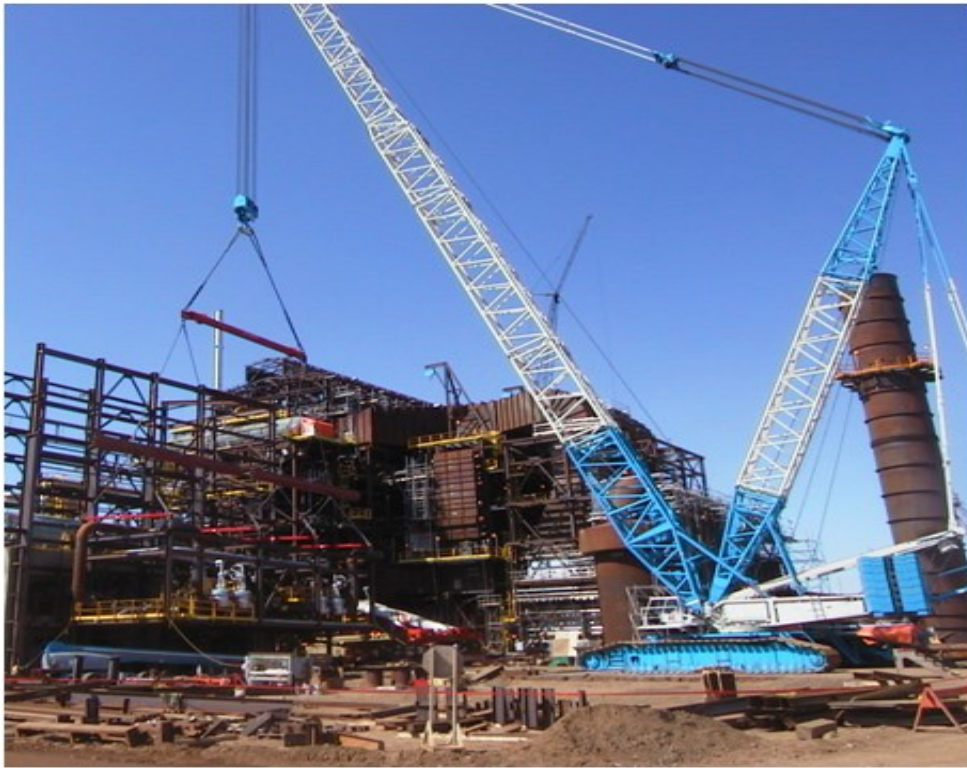
Figure 3-1 Pick-and-swing crane operation
