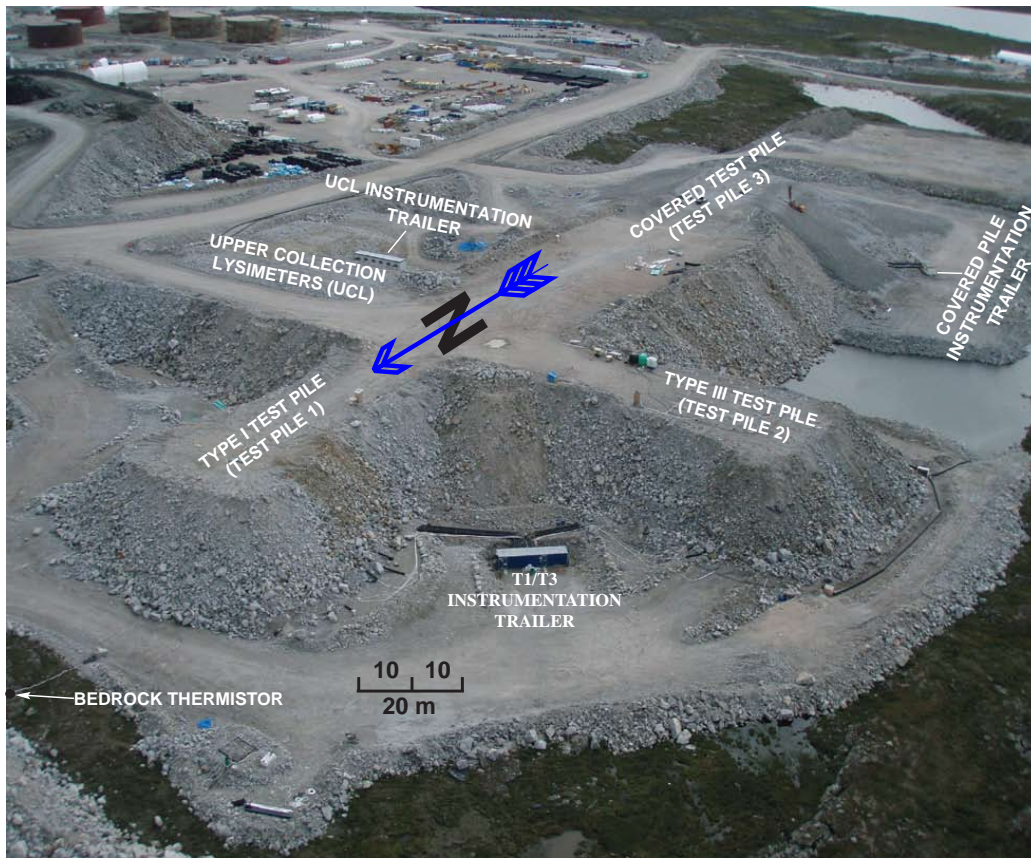
Figure 1.3: Aerial view of the test piles at Diavik diamond mine.
