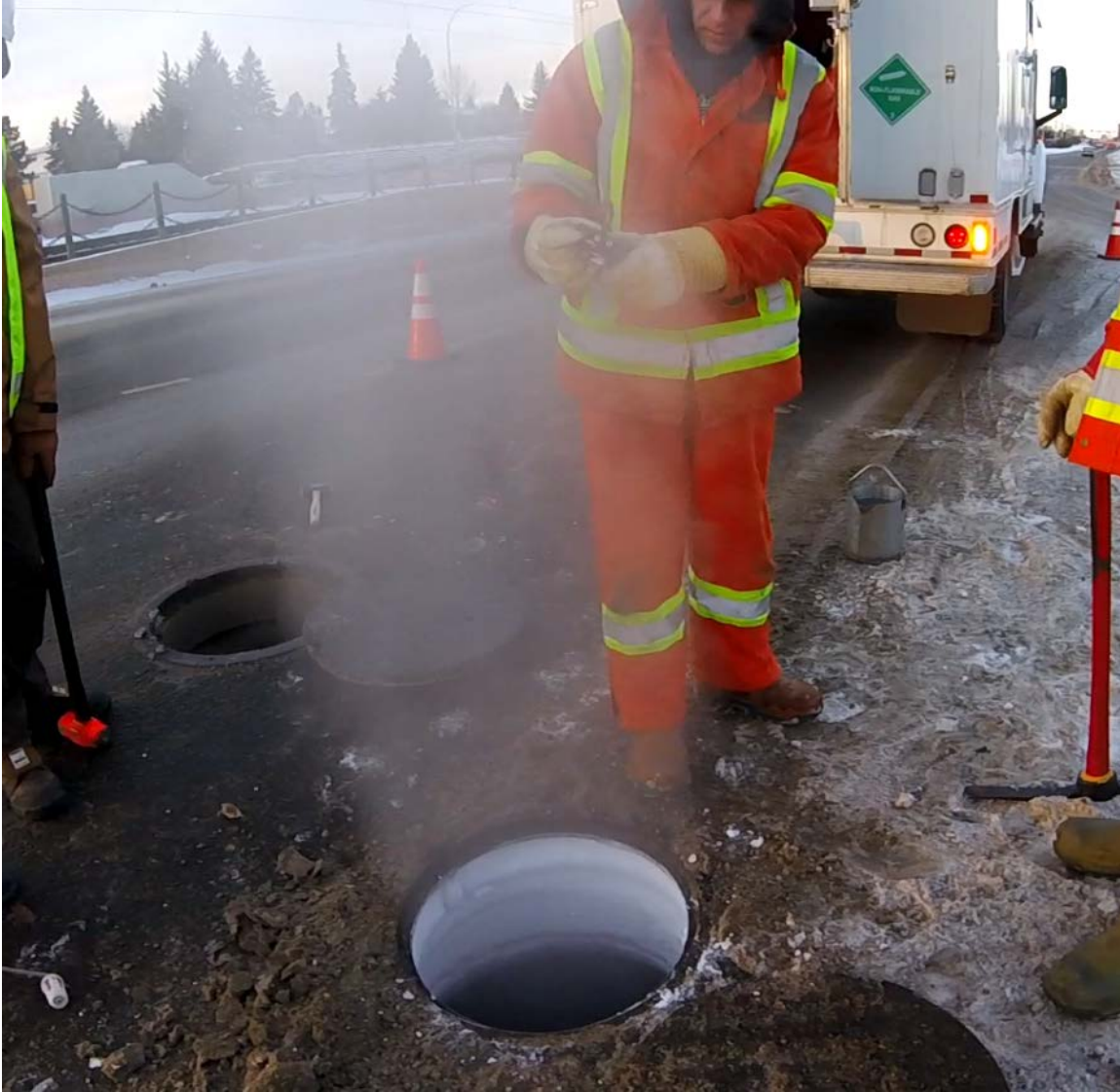
Figure 1-1 Photo of the air flowing out of the manhole due to a high pressure in the sewer system.
