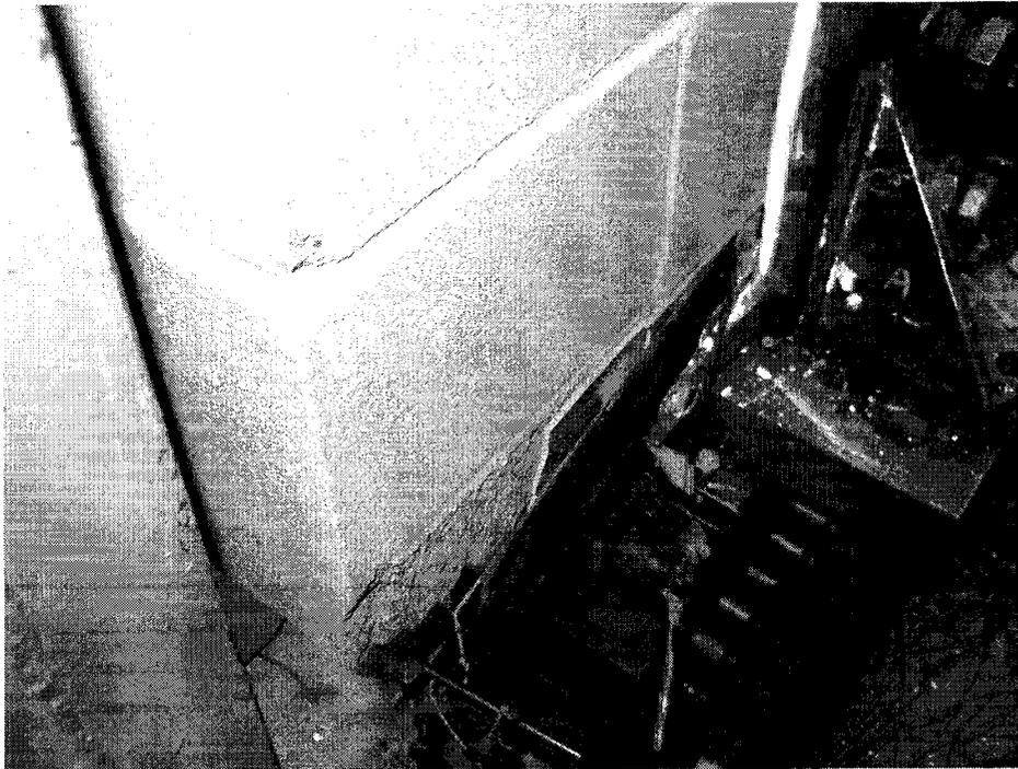
**Image 4-15 Peeling off at the End of Beam 5**
