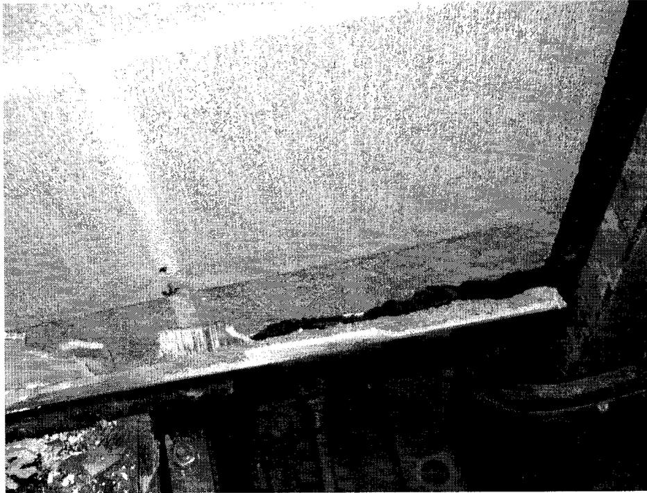
**Image 4-20 Peeling off at the End of Beam 6**
