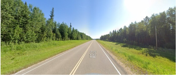
Figure 69. Road Section (2) – High Vegetation Density on Both Sides of Frame 1100
