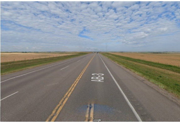
Figure 92. Environment for Road Section (5) at the 0.5 km Mark
