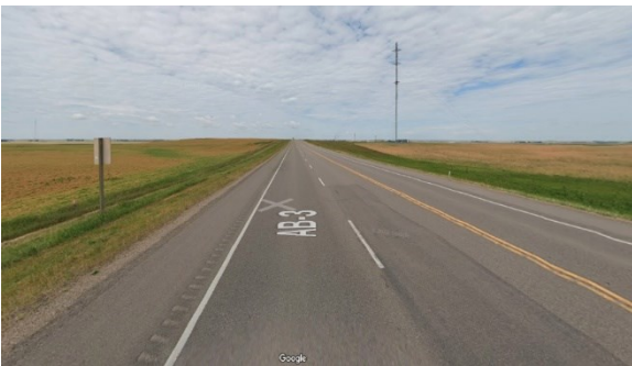
Figure 94. Environment for Road Section (5) at the 1 km Mark
