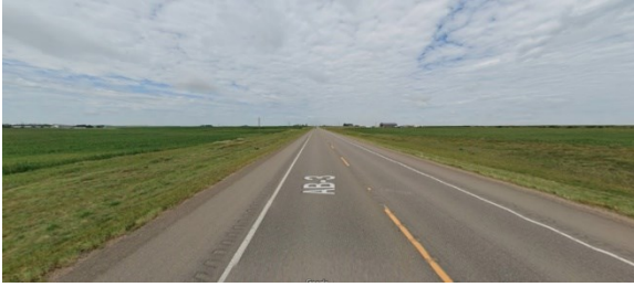
Figure 87. Environment for Road Section (4) at the 0.5 km Mark
