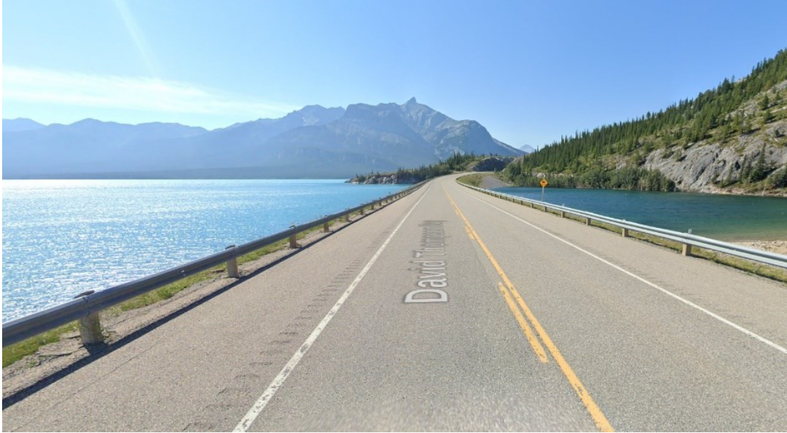
Figure 112. Waterbody Along Road Section (9)
