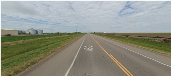
Figure 89. Environment for Road Section (4) at the 1.7km Mark
