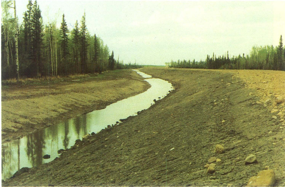
PLATE 3. The West Interceptor Ditch (Station 5) before hydroseeding and fertilization. May, 1977.
