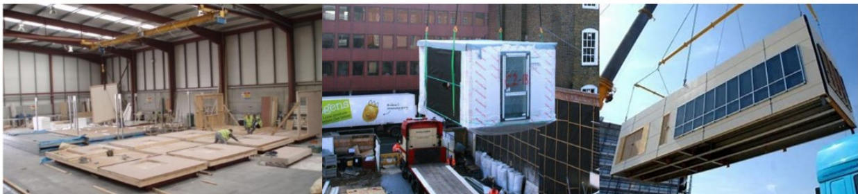
Figure 2. 2. Offsite Construction Method (Source: Iko team, 2024)
