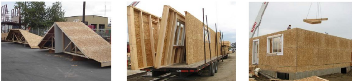
Figure 2. 11. Pictures of Prefabricated Panels (Mah, 2011).
