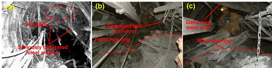
Figure 4.30 Pictures showing severe failure of steel arches, damaged belt conveyer, rockfall, and floor heaving in deep roadways after rockbursts ((a) is from Horyl and Snuparek, 2012; (b) and (c) are from Mutke et al., 2009).
