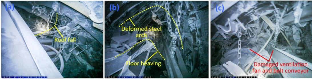
Figure 3.4 Field observations of rockburst damage of the “5.5” rockburst event (after Jastrzębska Spółka Węglowa S.A. Group, 2019).
