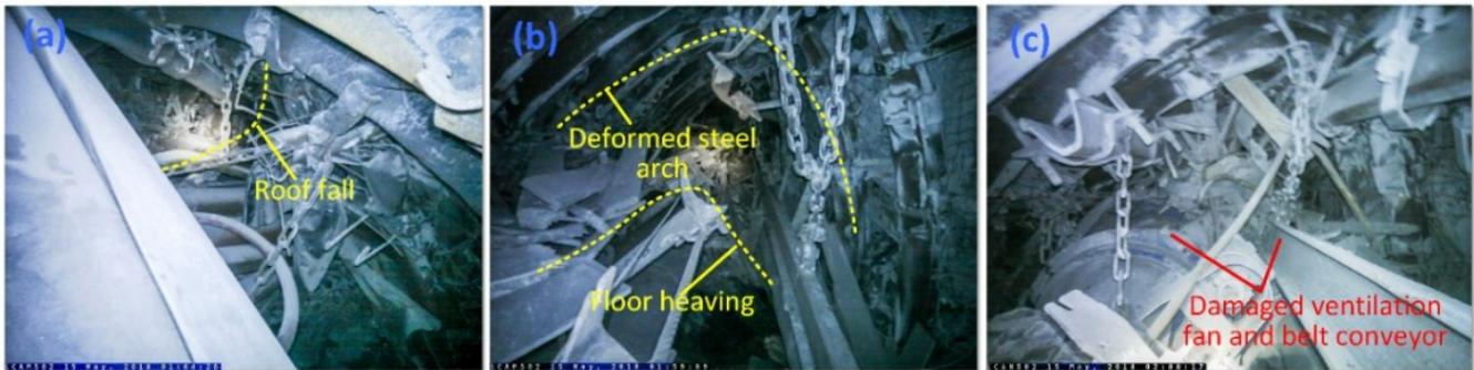
Figure 6.16 In situ observations of rockburst damage caused by the “5.5” rockburst event (after Jastrzębska Spółka Węglowa S.A. Group, 2019).
