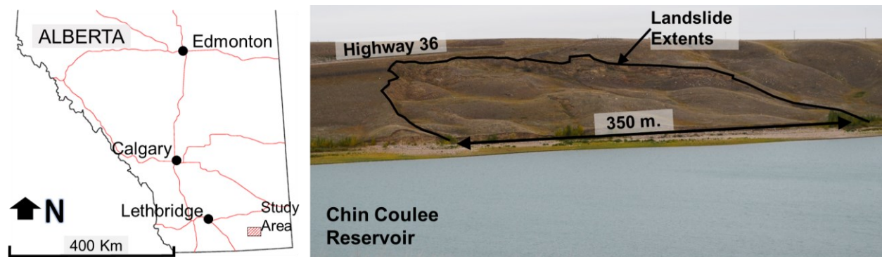
Figure 4.2 Chin Coulee landslide location and geometry characteristics
