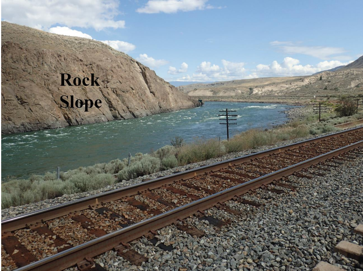
Figure 3-8 Rock slope along the West side of the Thompson River across from the Ripley Landslide
