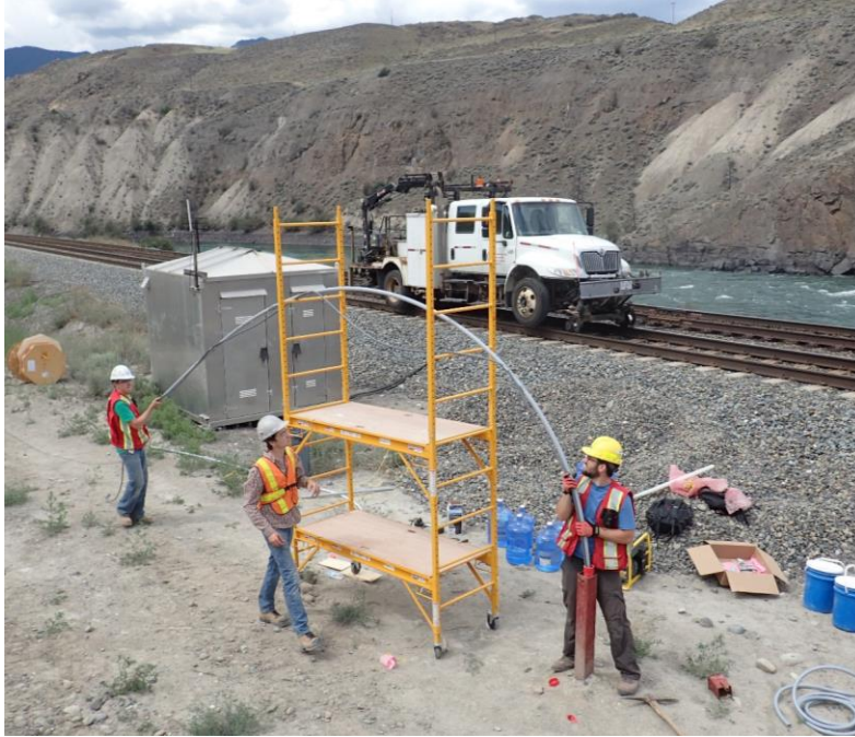
Figure 3-14 Installation of ShapeAccelArray into BH15-04 in July 2015
