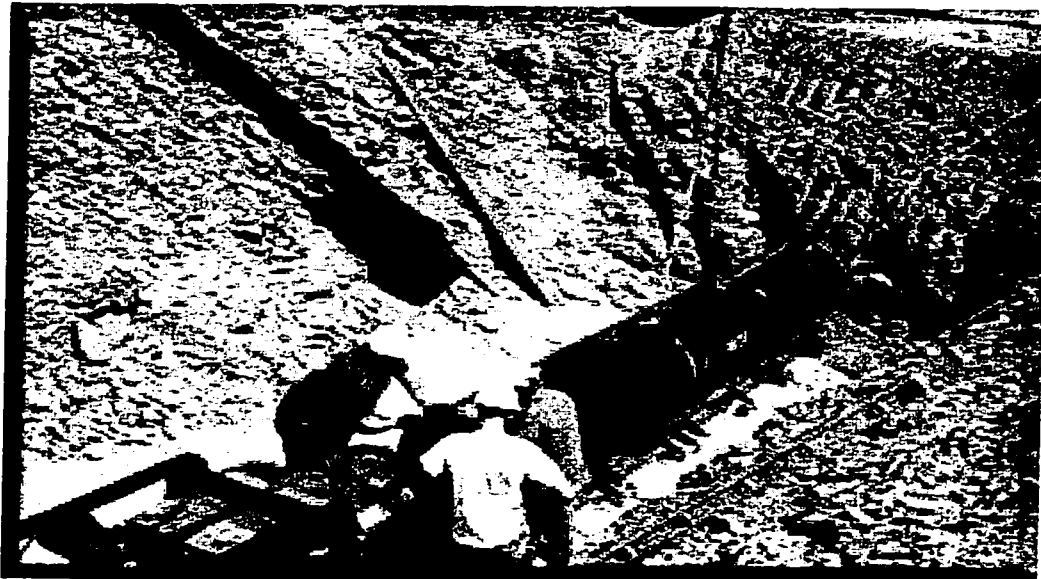
Figure 2-4 Auger Boring Set-up
