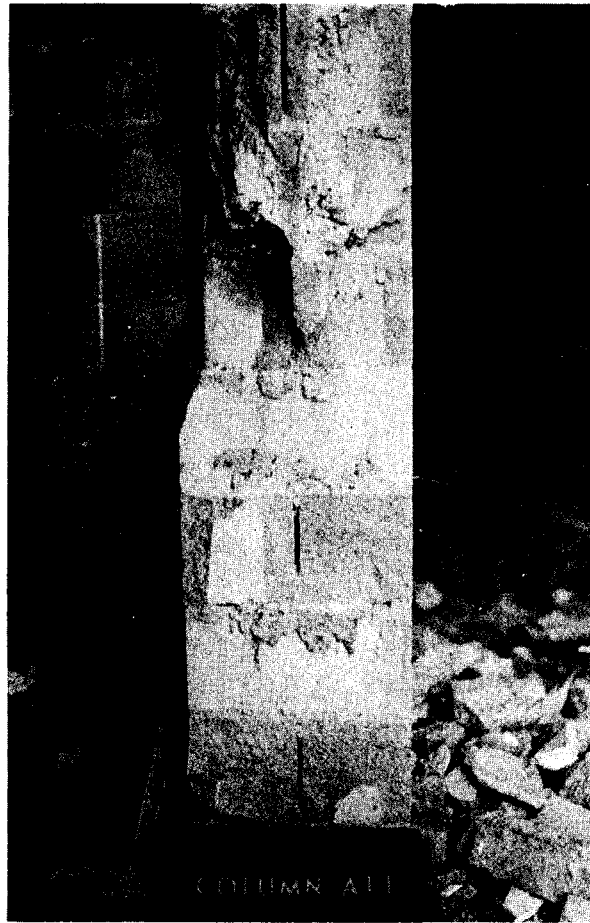
PLATE 5.1 FAILURE OF COLUMN BY VERTICAL SPLITTING
