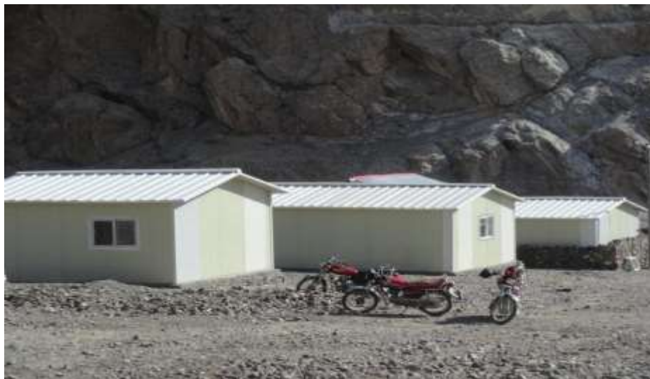
Figure 10. Pre-fabricated model of shelter conceived and allocated by the Aga Khan Agency for Habitat to the 260 earthquake-affected families in Chitral during 2015-2016
