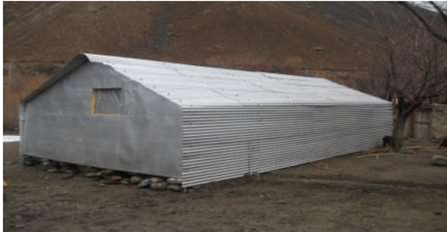
Figure 9. Old design of the shelter allocated by the Aga Khan Agency for Habitat to the 85 disaster-affected families in 2010
