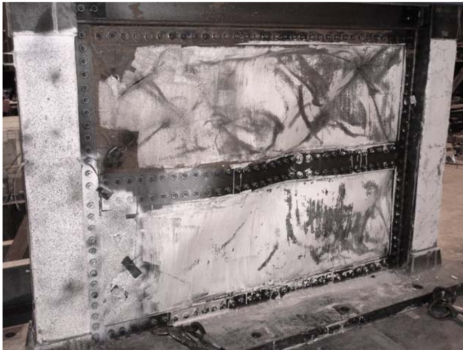
Figure 5.8: First story of the specimen at the end of the test
