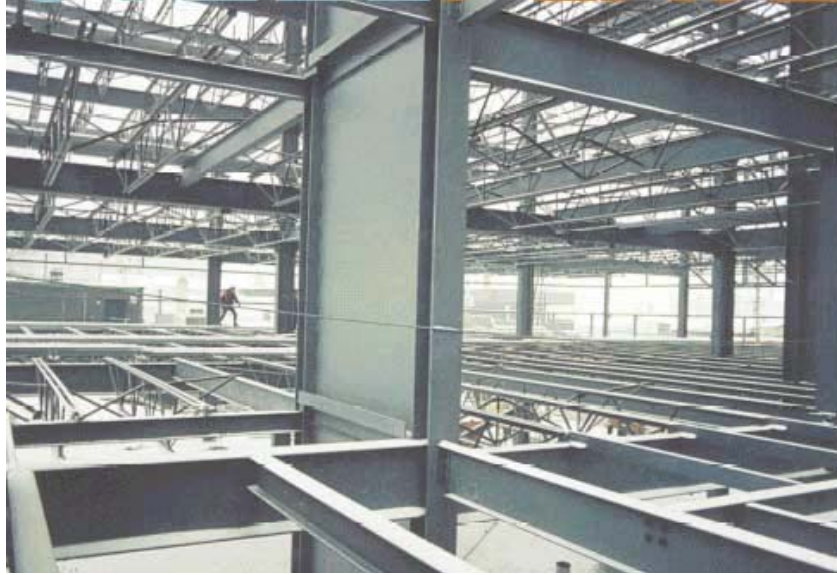
Figure 1.1: Typical steel plate shear wall (Photo courtesy of Canam Group)
