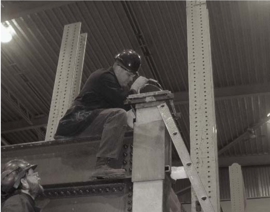
Figure 4.18: Grouting of the remaining gap under the cap plate
