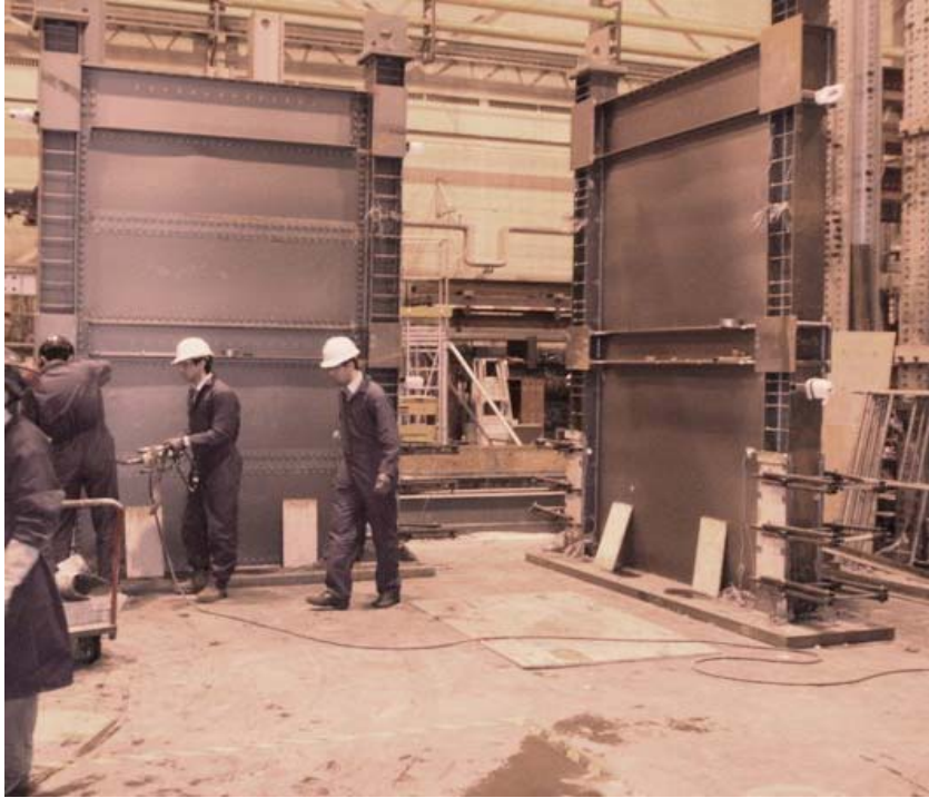
Figure 4.16: Formwork before the first cast of concrete in columns
