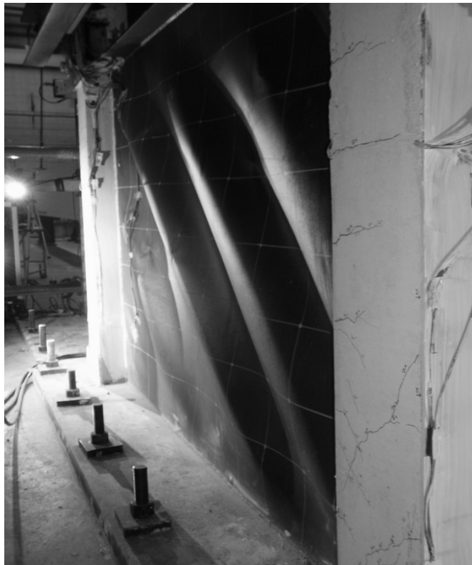
Figure 1.2: Development of tension field in post-buckling stage in steel plate shear wall
