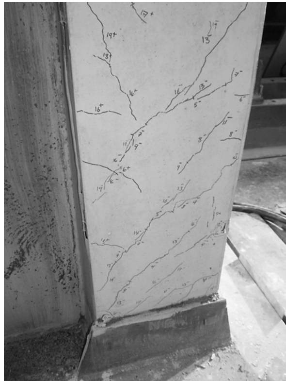
Figure 6.4: Bottom part of east face of the north column in cycle 19
