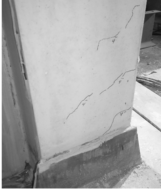
Figure 6.1: East face of north column in cycle 4
