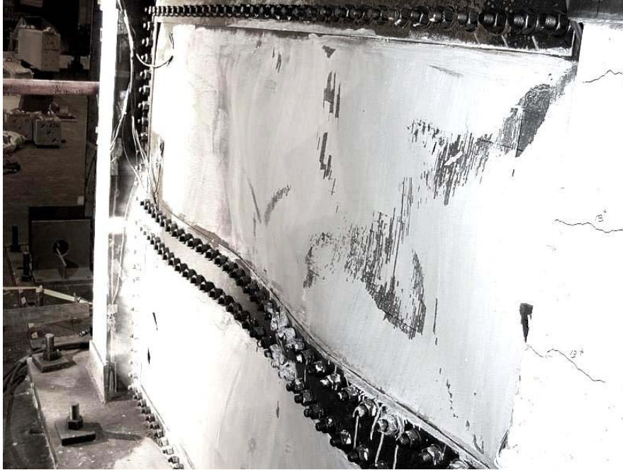
Figure 5.3: Yield lines in the infill plate of the first story during cycle 15
