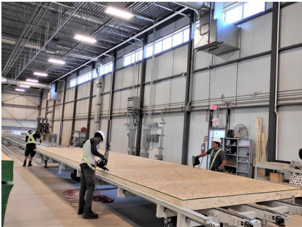
Figure 4-4. Sheathing station (manual nailing of sheets for exterior walls)
