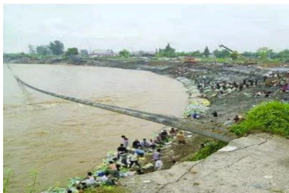
Figure 1-3 Spanning pipeline caused by flood [36].
