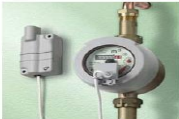
Figure 49: Smart Water meter with data logger
