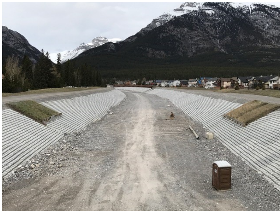
Figure 2-2 Cougar Creek debris flood infrastructure
