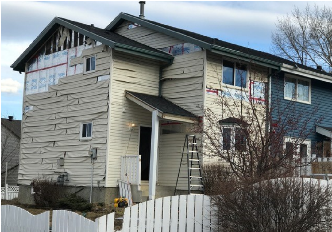
Figure 3-4 Vinyl siding damage, Fort McMurray, AB
