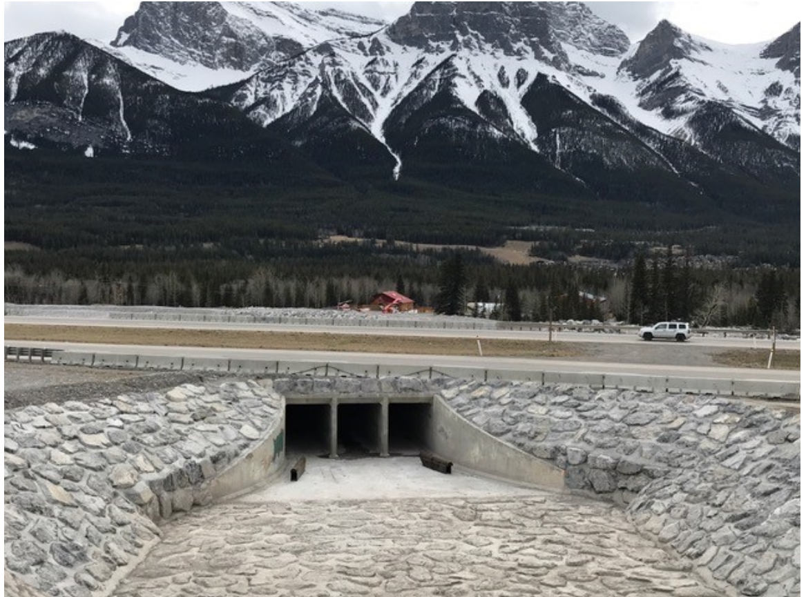
Figure 3-3 New Cougar Creek culvert in Canmore, AB
