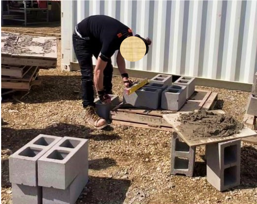
Figure 12: The bricklayer performed laying blocks to make a 1 \times 5 block line
