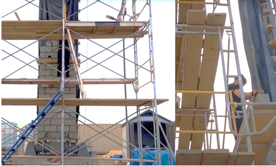
Figure 13: The bricklayer performed laying blocks to make a 1 \times 3 block line
