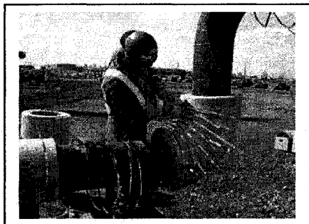
(f). Pipe insulation
