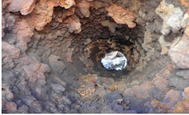
Figure 3-2: Inside of the tuberculated pipe (Wassam, 2015)
