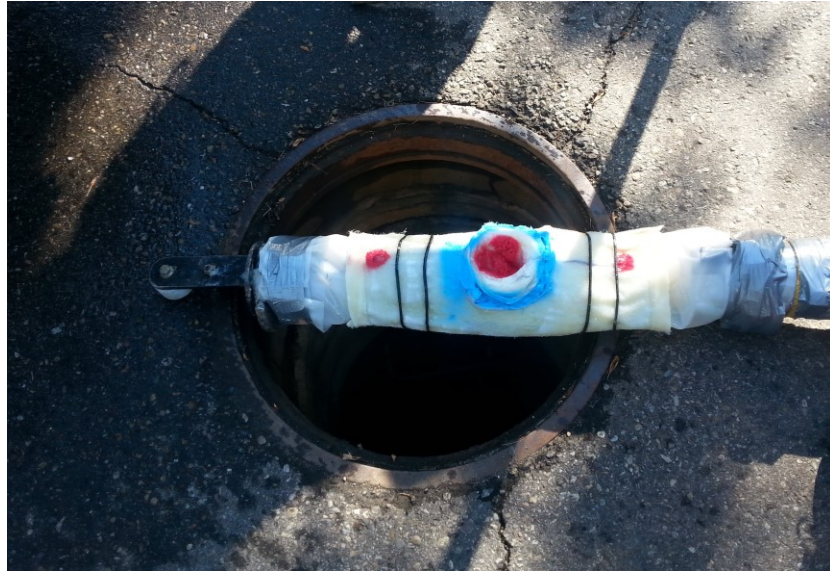
Figure 2-11: Resin-impregnated, single-piece lateral and main connection liner assembly prior to installation (site visit at an installation in Edmonton, Alberta)
