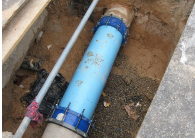
Figure 3-7: Lined pipe sections connected by PVC pipe (Matthews et al., 2015)
