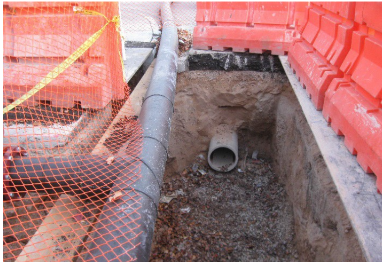
Figure 3-4: Access pit with pipe removed (right) and bypass (left)(Matthews et al., 2015)
