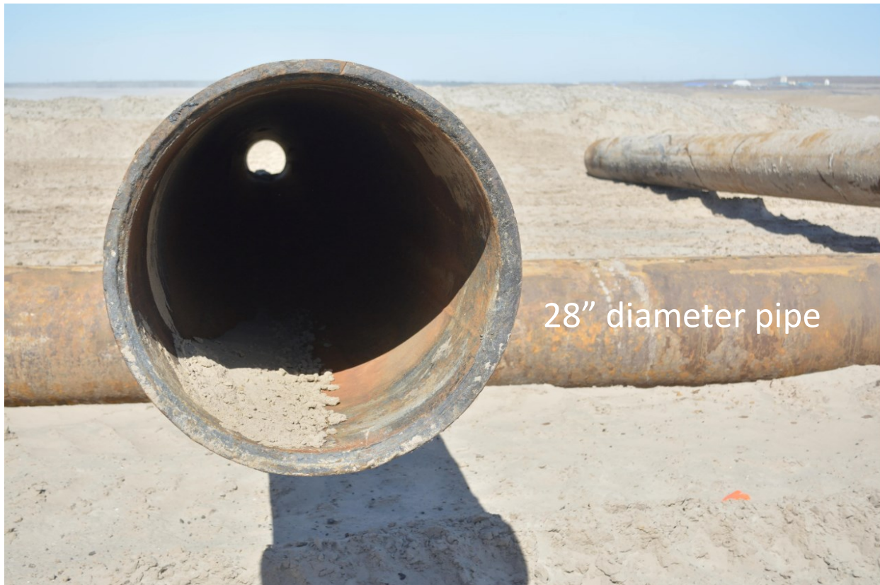
Figure 10. Photo of out of service friction fit pipe.
