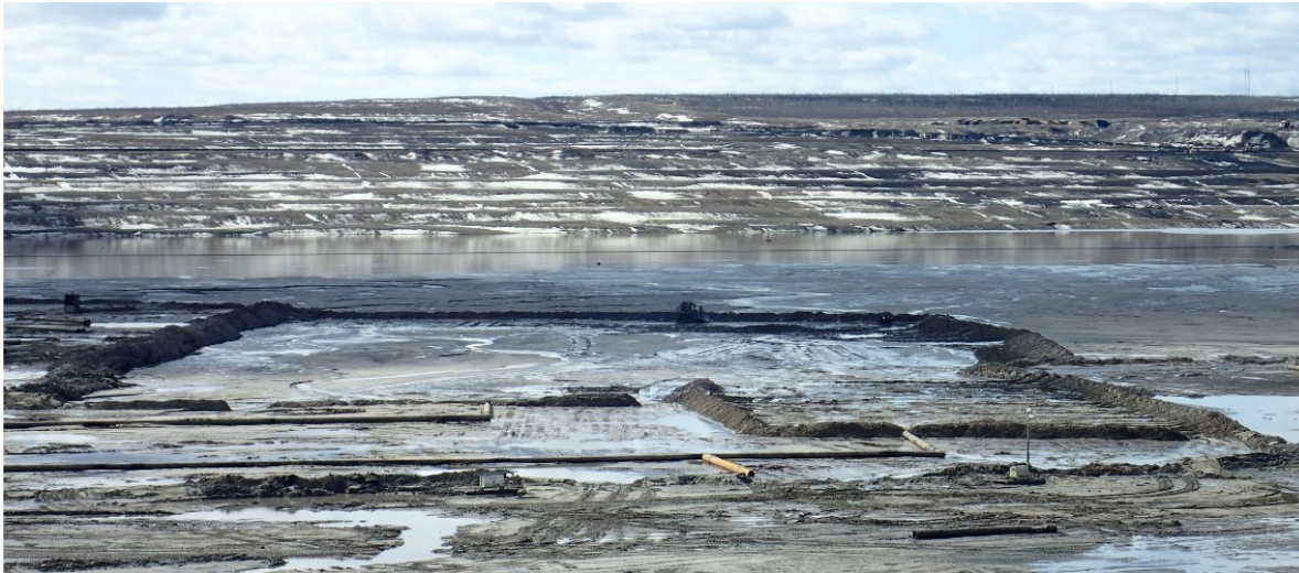
Figure 5. Cell construction in the tailings discharge area at an oil sands mine.
