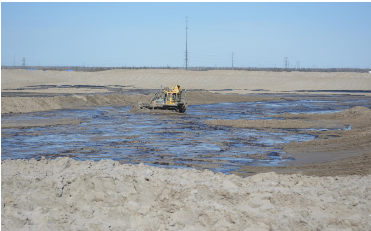
Figure 7. Bulldozer compacting sand in the tailings discharge area.
