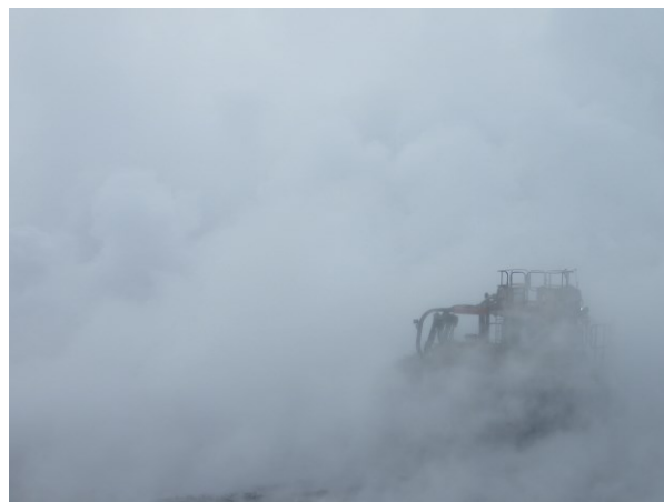
Figure 43. A bulldozer shrouded in steam in the tailings discharge area.
