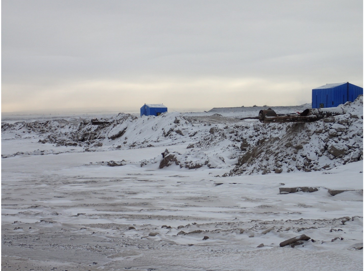
Winter Photo (g), View of tailings discharge area and end of line device (right) while not in use; erosion on ground below end of line device.
