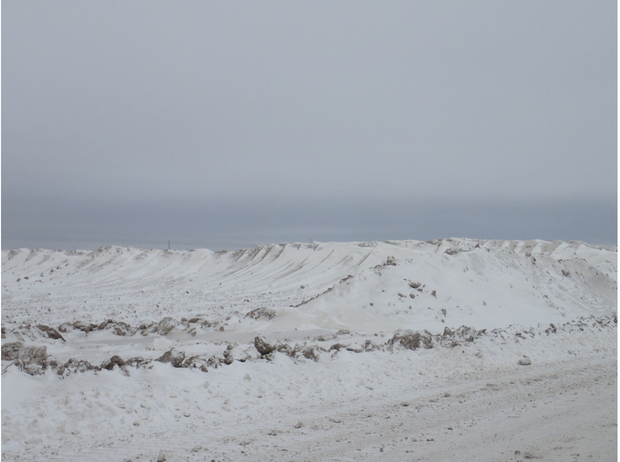
Winter Photo (b), View of snow-covered eroded slopes of tailings dam.
