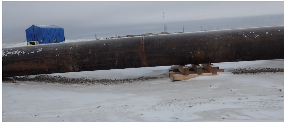
Figure 18. Example of a pipeline elevated on blocking for a full 360° view.
