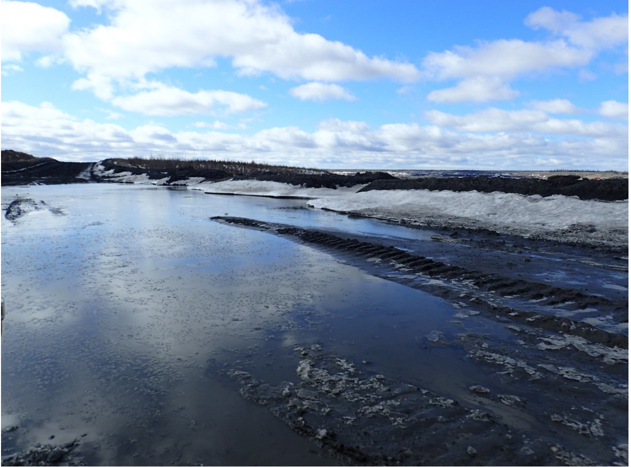
Spring Photo (e), Standing water on road with ice melting on the side.
