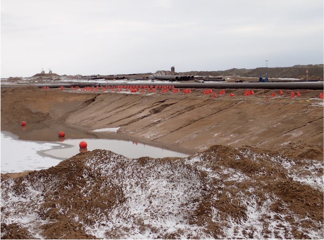
Spring Photo (b), Seepage from face of dyke with ice and standing water at the toe.
