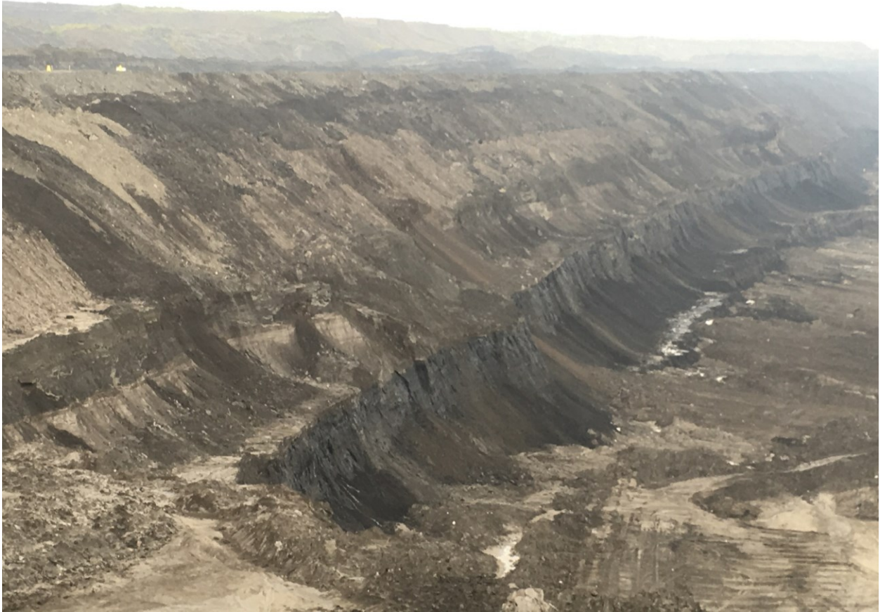
Summer Photo (a), View of the open pit (~30 m deep). Steep slopes (~55°) typical of mining operations. A failed slope can be seen (top) at an inactive pit area
