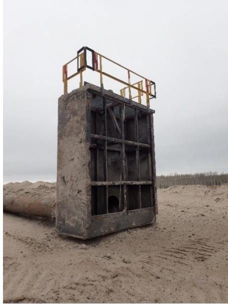
Figure 19. Out of service spill box with handrails installed.
