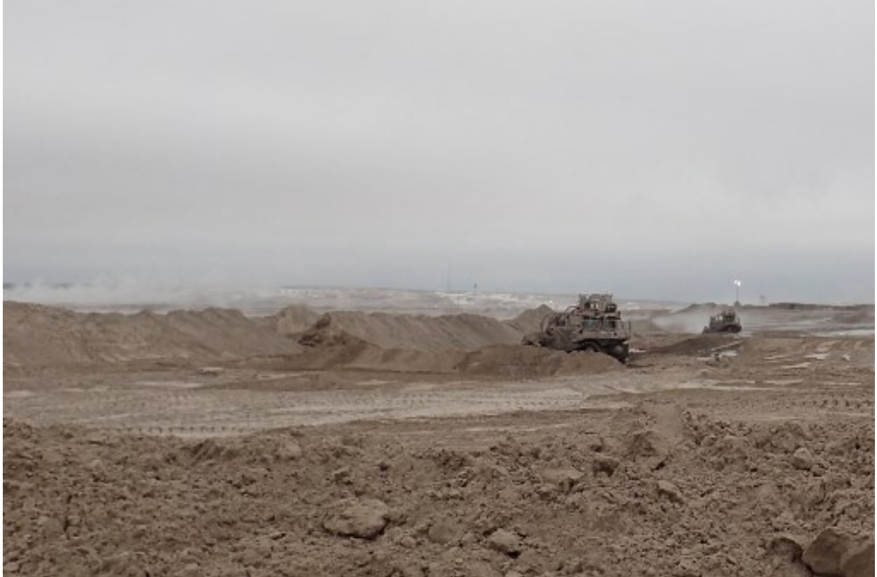
Summer Photo (b), Bulldozer creating steep cell walls in tailings discharge area.
