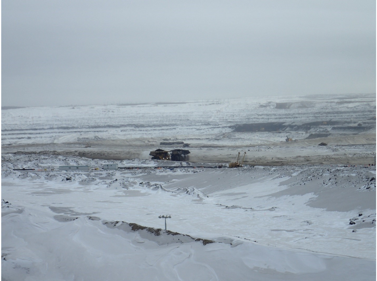
Winter Photo (a), View of the open pit. Steep slopes ( \sim 55^\circ ) typical of mining operations and snow-covered benches.
