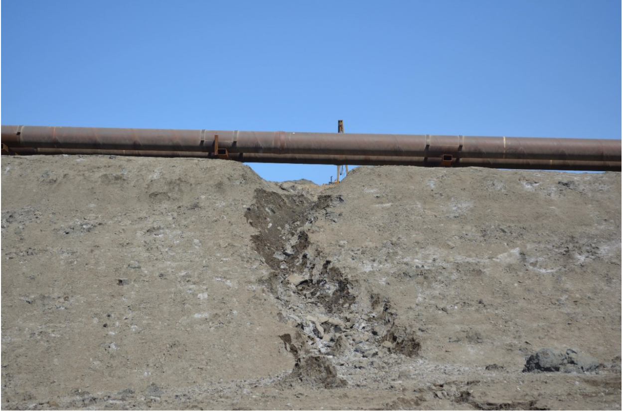
Spring Photo (g), Slope in the tailings discharge area with pipeline and erosion features.
