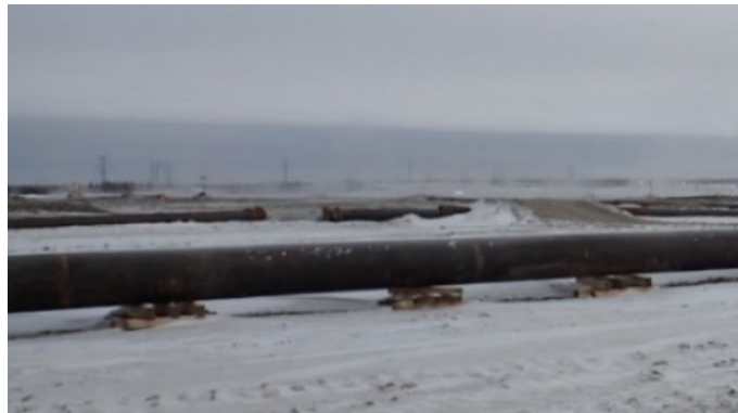
Figure 33. Pipelines elevated on blocking.
