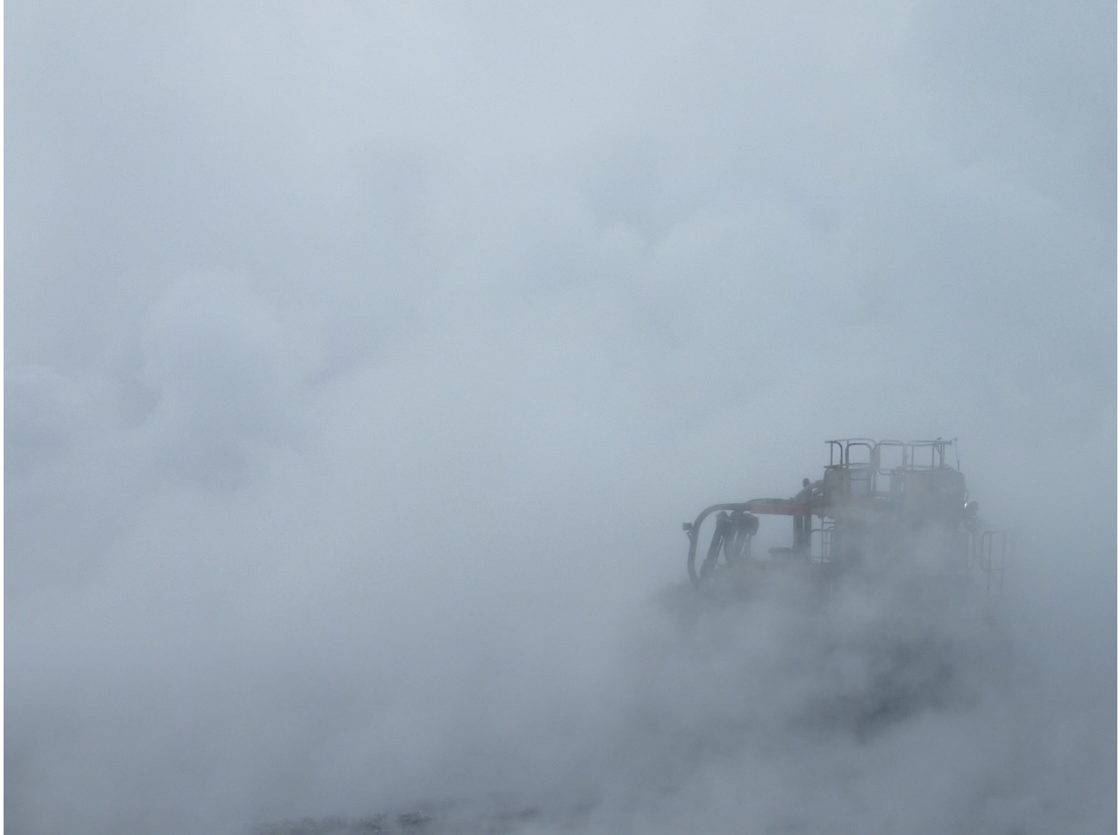
Winter Photo (d), Close-up of bulldozer in soft ground at tailings discharge area with steam from hot tailings discharge.
