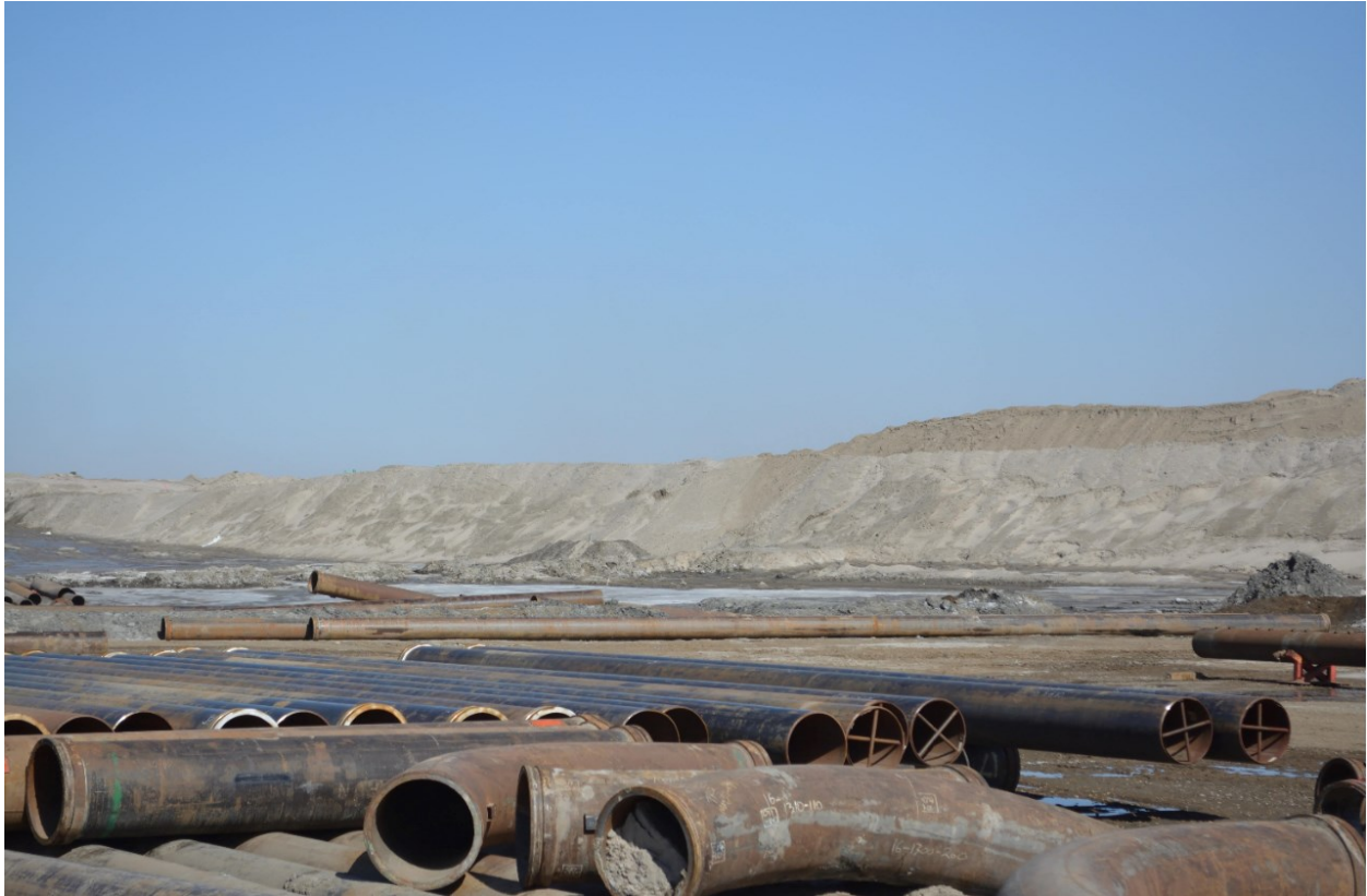
Spring Photo (a), Seepage at the toe of dyke with some unstable areas (middle) seen on the face.
