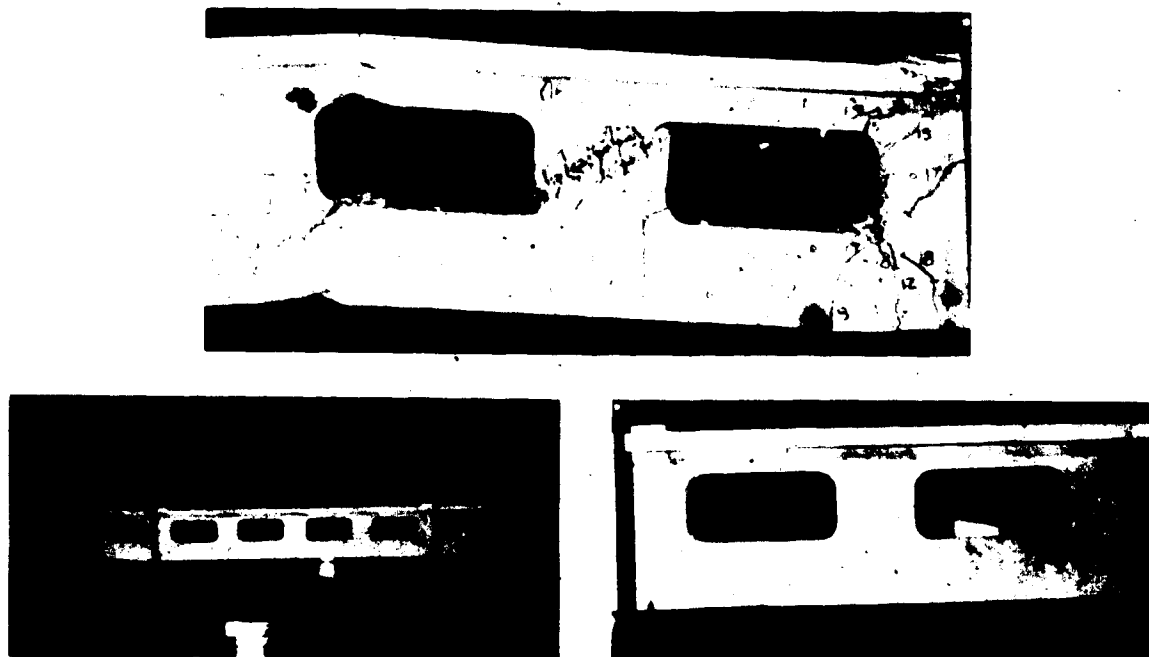
FIGURE 4.114 CRACKING AND FAILURE PATTERN OF BEAM 6-16-6
