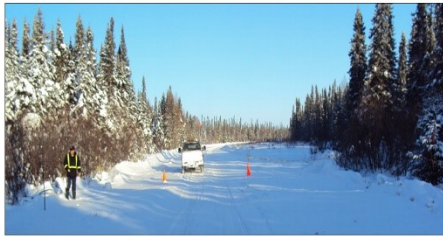
312-KM Ice Road Connecting First Nations Communities of James Bay
