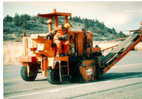
(i) Pothole edges are straightened up
