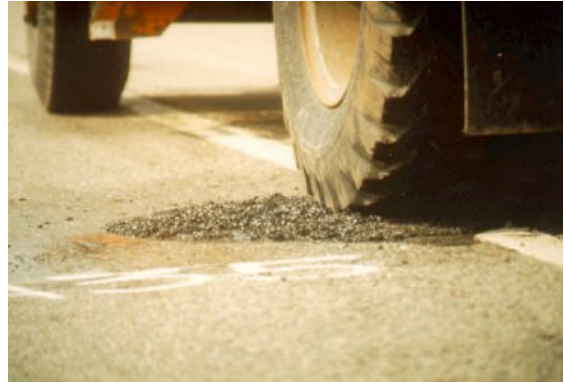
(ii) Compacting using truck tires
