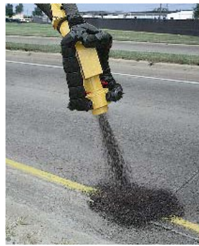
(ii) Blowing asphalt and aggregate into pothole
