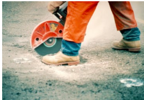
(i) Pothole edges are straightened up
