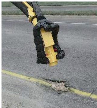
(i) Blowing water and debris from the pothole
