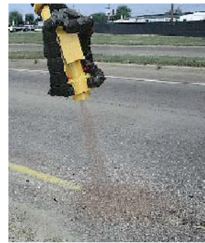
(iii) Covering patch with dry aggregate
