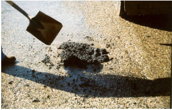
(i) Placing material into pothole
