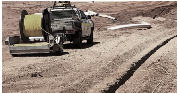
Figure 3. Installation of fibre optic cable at a TSF site
