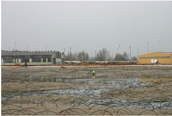
Figure 18. Tubes after installation, ready to be connected
