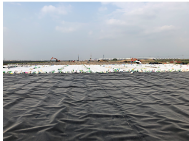
Figure 7. Installation of the sealing liner in a liner vacuum project
