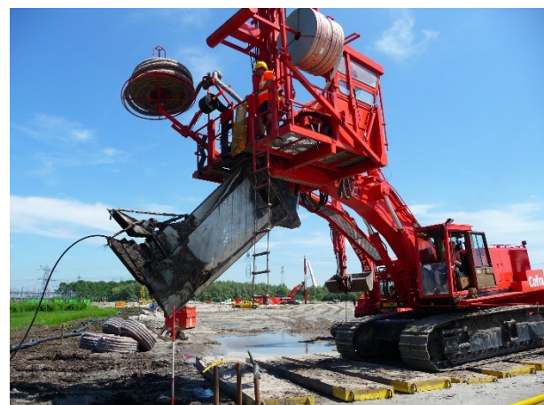
Figure 10. BeauDrain installation equipment
