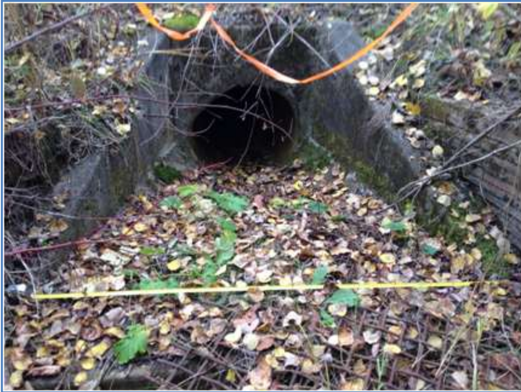
Figure 7a – Broad crested weir and culvert on outlet channel from Jackfish Lake.
