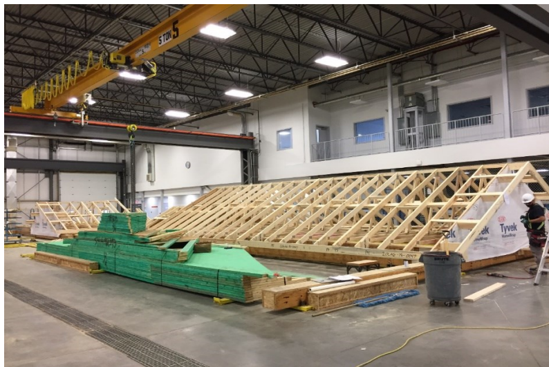
Figure 1.4. Roof production station (source: ACQBUILT Inc. 2019).
