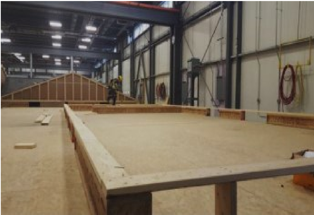
Figure 1.5. Roof jig platform (source: ACQBUILT Inc. 2019).
