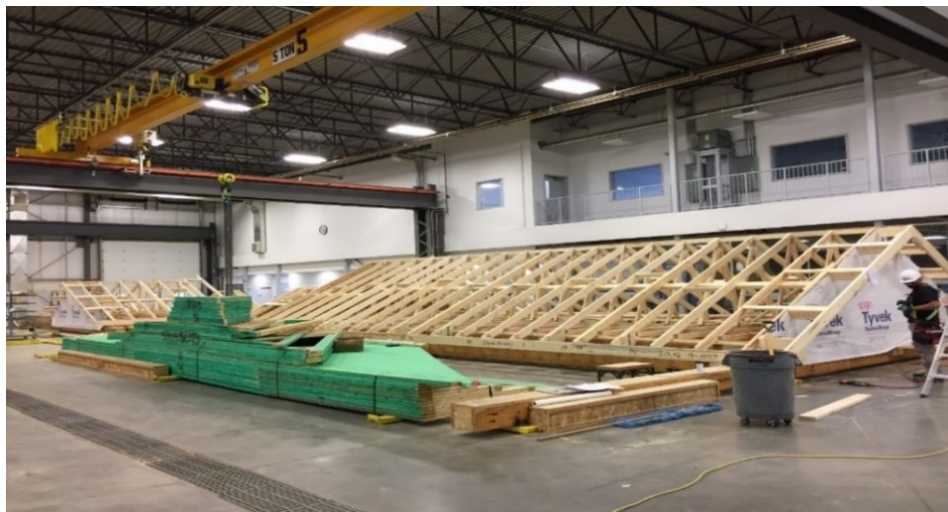
Figure 3.2. A roof production line (ACQBUILT Inc. 2019).
