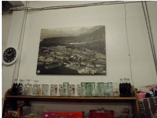
Figure 2-8: Photograph of a mill site during mill era at the Youbou Lanes bowling alley (Image: C Lyon)
