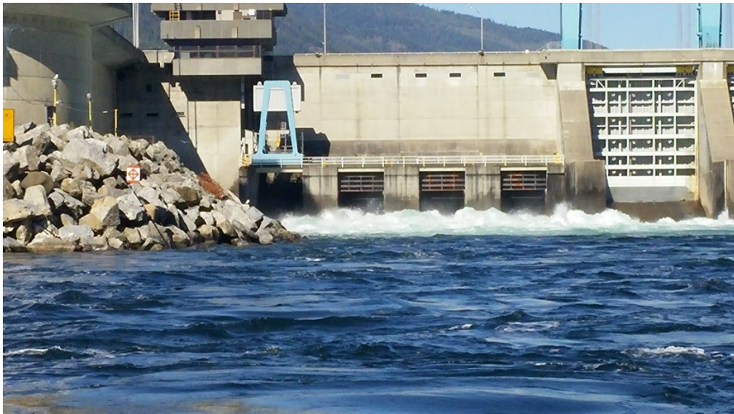
Figure 41: SL5,6,7 in operation with typical surface turbulence
