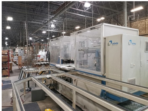
Figure 3-6. Auto-corner cleaning station
