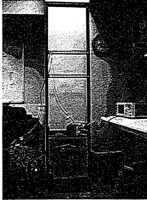
Figure 2.9: Rack housing the patch panels
