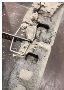
Figure C.14: T-PV.CN-1 connector condition after testing and veneer removal
