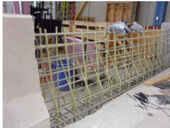
Figure 2.14: Doweling technique showing hole layout and photograph of planted reinforcement (El-Salakawy et al. 2014).
