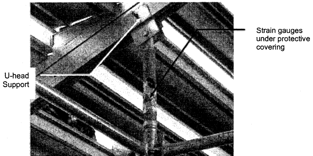
Figure 3.10. Strain gauges mounted on U-head post
