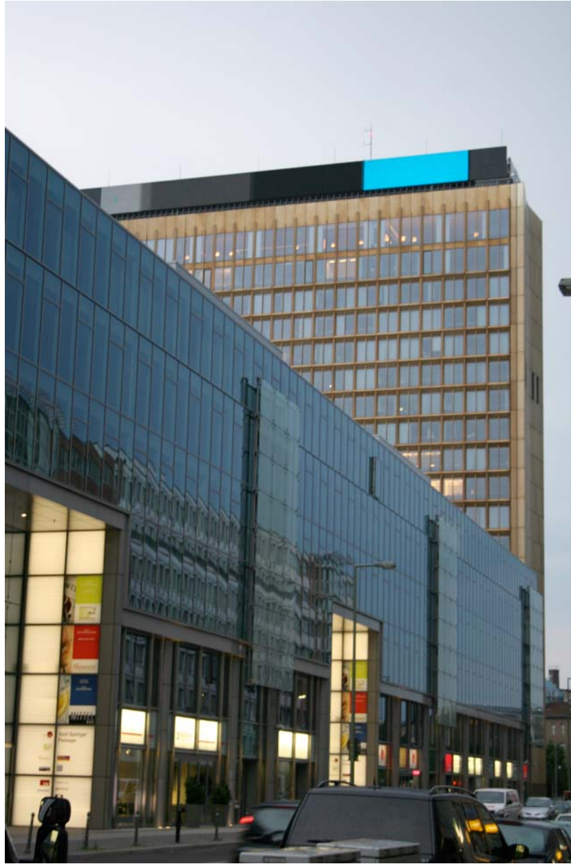
Figure 20 Springer Publishing buildings on Kochstraße in Berlin 2007
