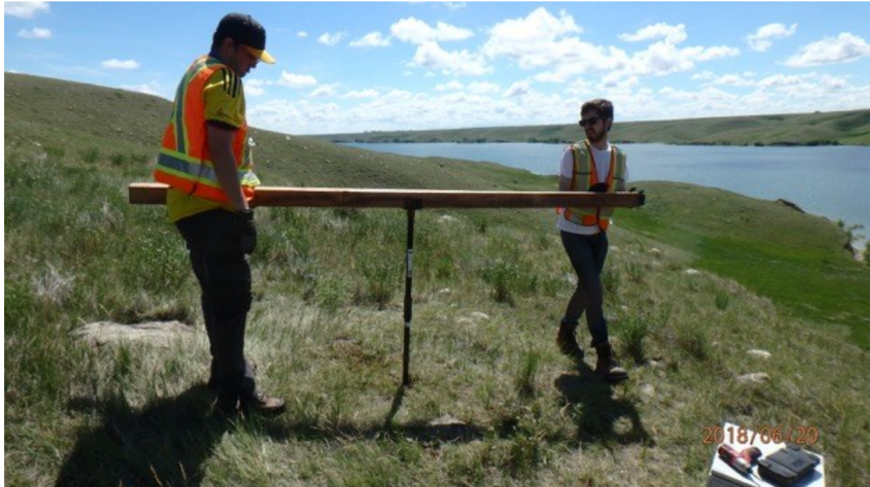
Figure 4-2: Chin Coulee GPS deck screw pile installation (Hong 2018)
