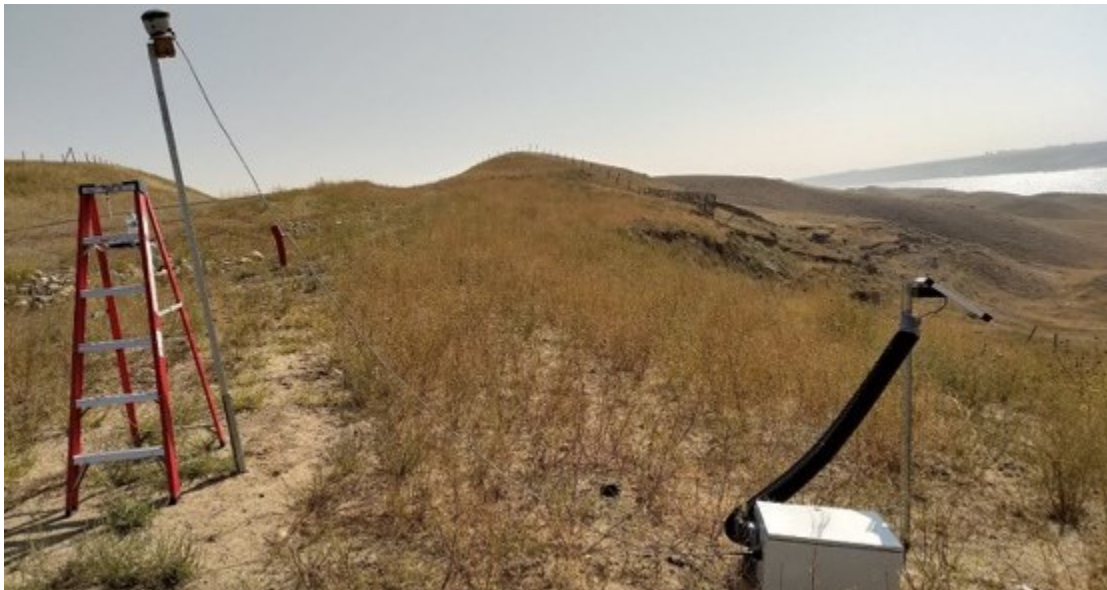
Figure 4-6: Headscarp GPS unit at Chin Coulee after external antenna relocation and raised GPS unit
