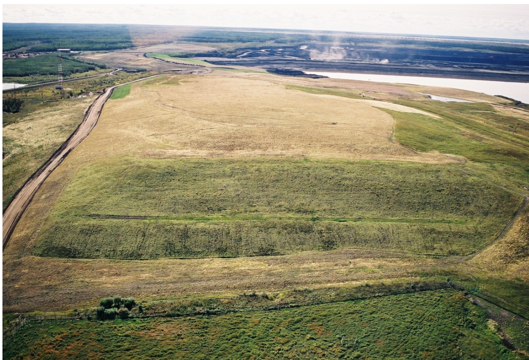
Figure 2-4. East slope several years after reclamation repairs (2001).
