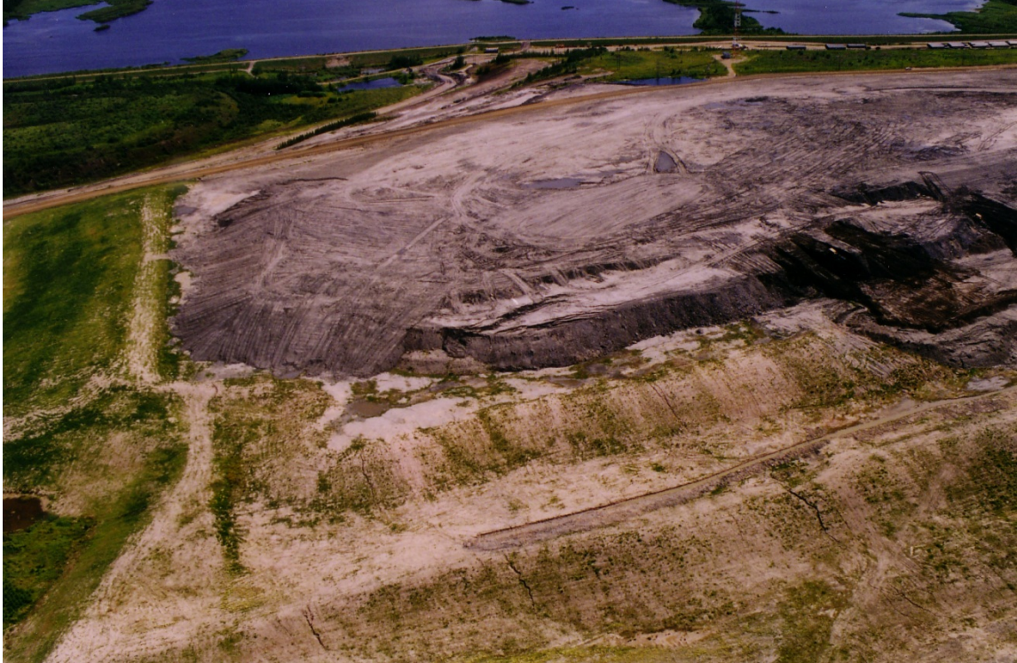
Figure I-4. Aerial view looking south during the construction phase of SBH. Photo taken between 1997-1998
