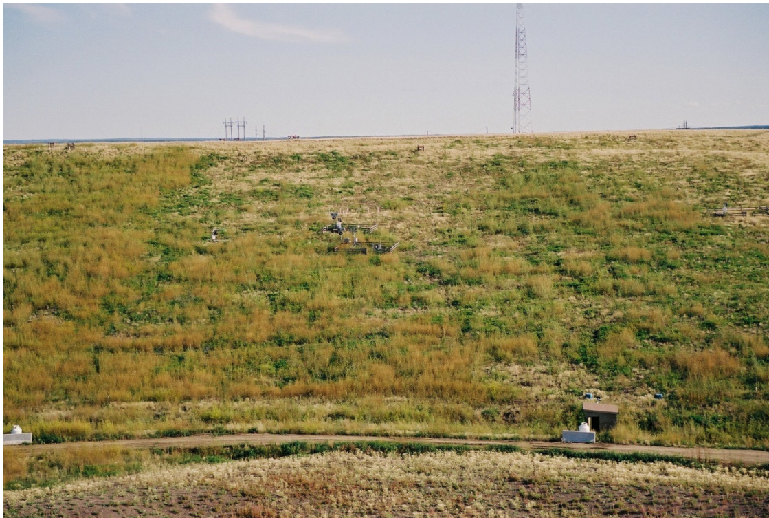
Figure I-19. Cover D2, note weir hut and weather station on the slope (2001).
