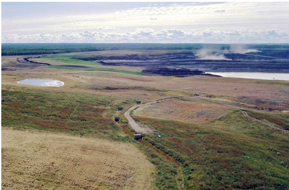
Figure I-8. Post-construction with view looking west (2001). Weirs D1, D2 and D3 of capping study are visible, as well as Peat Pond on the left.
