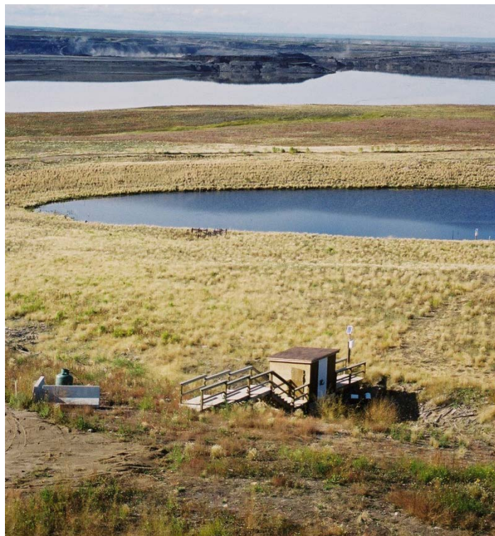
Figure I-11. Photograph of the main swale weir of SBH plateau, with Peat Pond visible in the immediate background followed by West-in-pit (2001).
