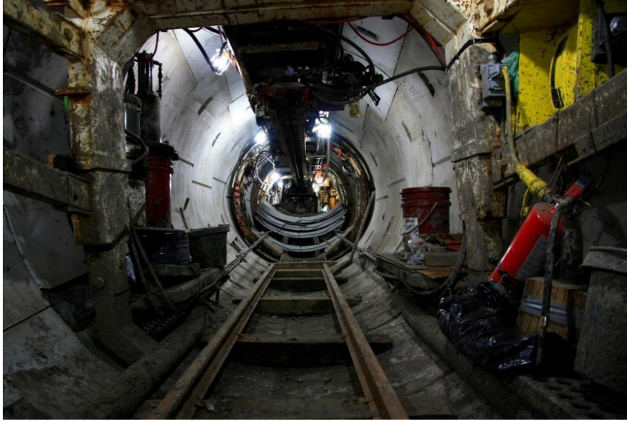
Figure 2-3: Inner view of a tunnel under construction by a TBM
