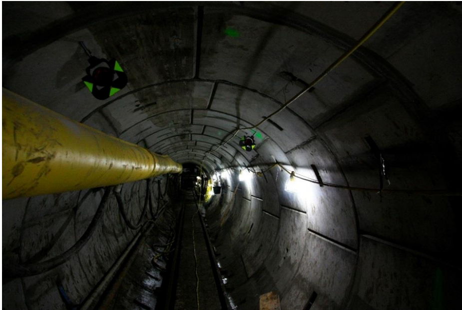
Figure 2-5: Typical environments inside a tunnel under construction
