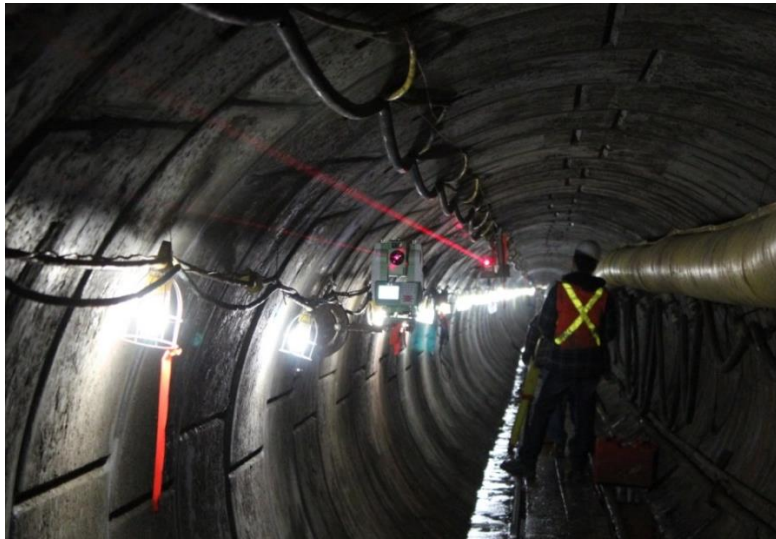
Figure 5-2: VLTB system under testing
