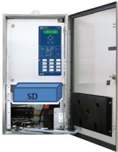
Figure 3.23 Installation of SD in local control cabinet of recloser
