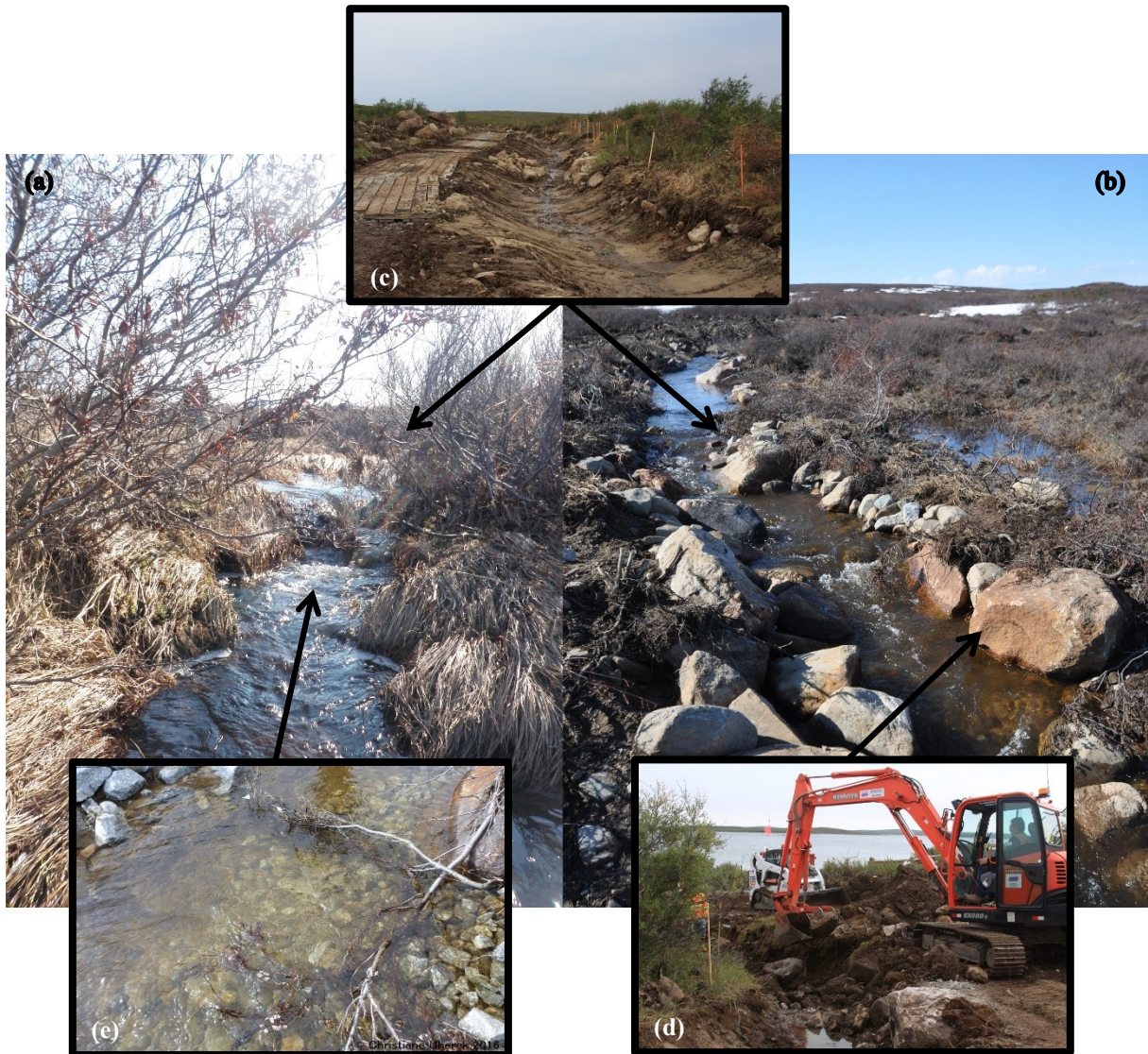
Figure 2.6: (a) West Island Stream (WIS) before manipulations; photo by M. Hulsman, taken on July 29, 2010, facing south, and (b) after manipulations; photo by C. Uherek, taken on May 31, 2013, facing south. (c) The channelization process, photo by C. Cahill, taken on August 18, 2012, facing south; (d) the boulder addition process, photo by C. Cahill, taken on August 18, 2012, facing north, and (e) wood pieces addition, photo by C. Uherek, taken on July 3, 2013, facing south.
