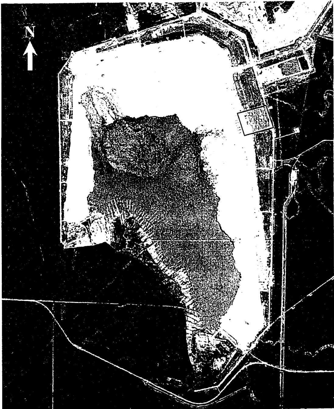
Figure 3.3 Location of Cell 32 on the SWSS (adapted from Syncrude Canada Ltd.)
