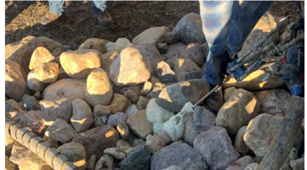
Figure 7. Polyurethane foam injection. Note excess foam at injection site.
