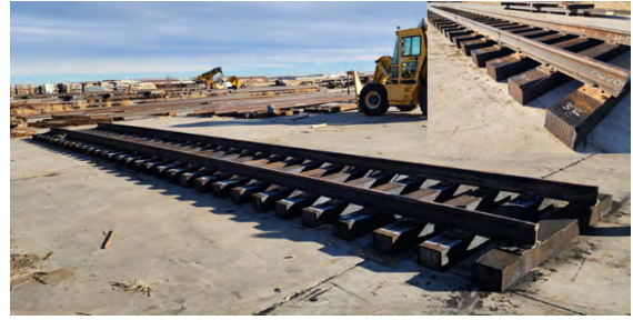
Figure 12. Track panel test setup.
