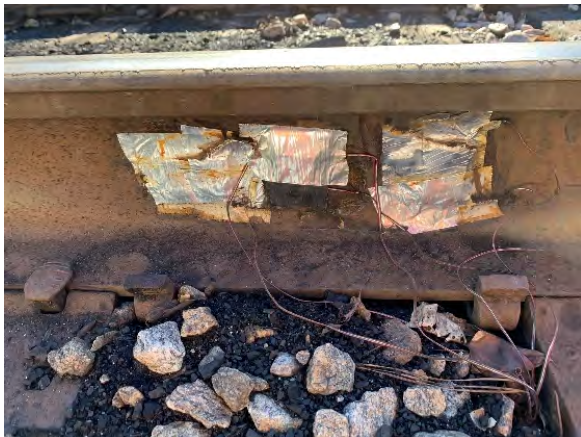
Figure 2. Strain gauges on rail
