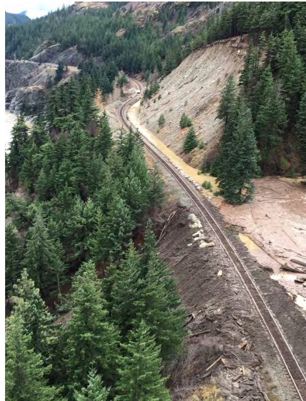
Figure 3. Debris (seen at far right of photo) filled the ditch and redirected drainage towards track east (top of the photo)
