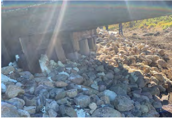
Figure 10. East abutment wall following project completion.
