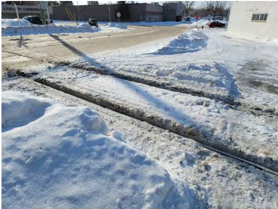
Figure 5. Grade crossing at 46.2802042, -96.0668825.
