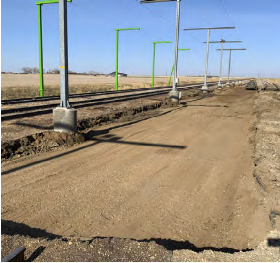
Figure 10. Base prepared for laying woven geotextile
