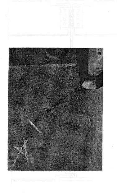
Figure 1.2 Crack Observed in the Web near the Coped Area of Bridge 51.1 Windermere Subdivision
