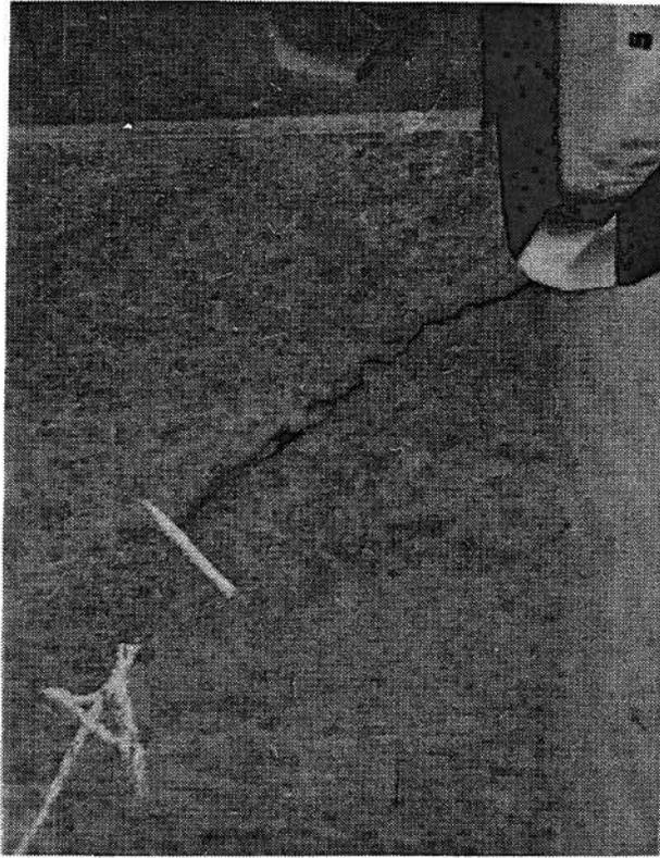
**Figure 1.2 Crack Observed in the Web near the Coped Area of Bridge 51.1 Windermere Subdivision**
