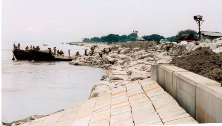
Figure 1.2: Image of sand-filled geotextile bags used for the Brahmaputra-Jamuna River in 1997 (near the Sirajganj town) [6]
