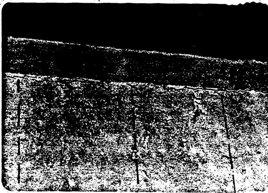
FIGURE 6.31 - Typical shrinkage cracks at bottom
