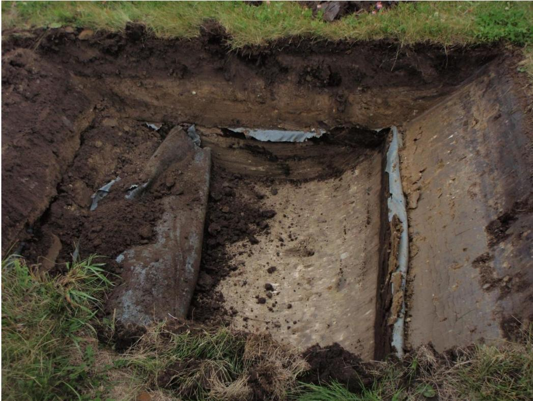
Plate 2.2 Removal of PVC liner and collection of nitrate impacted soil from below liner in nitrate fines landfill (September 15, 2010).
