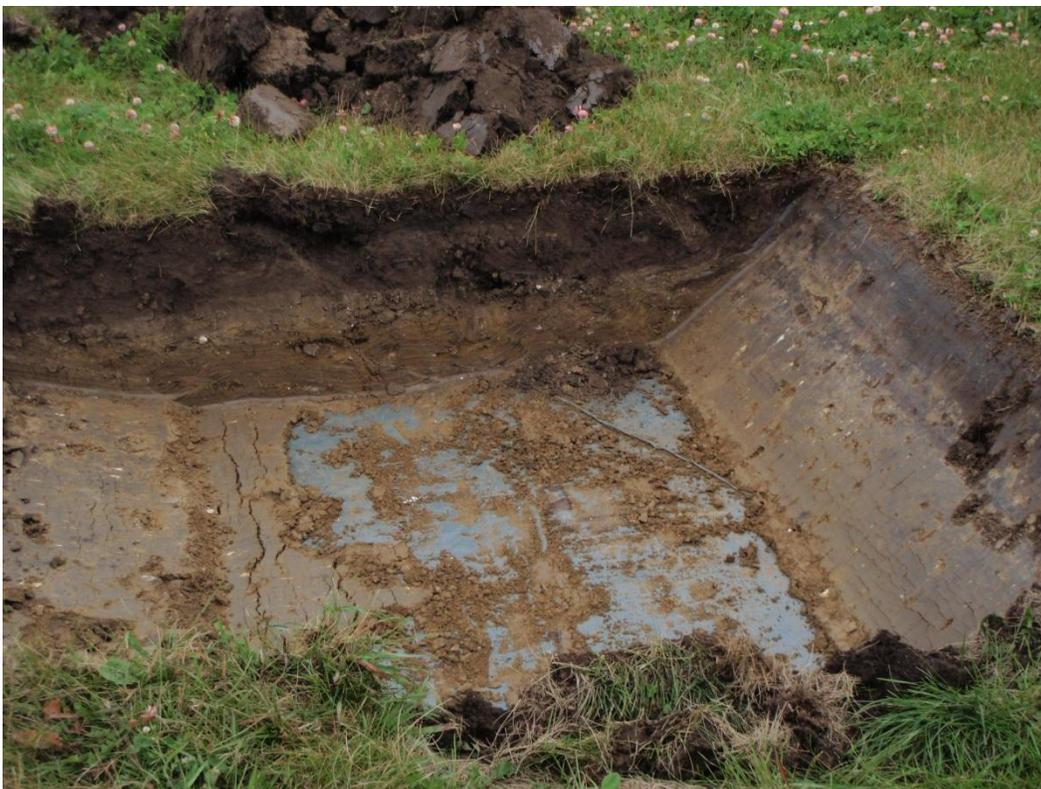
Plate 2.1 PVC liner exposed following stripping of vegetation and topsoil for collection of soil from nitrate fines landfill (September 15, 2010).
