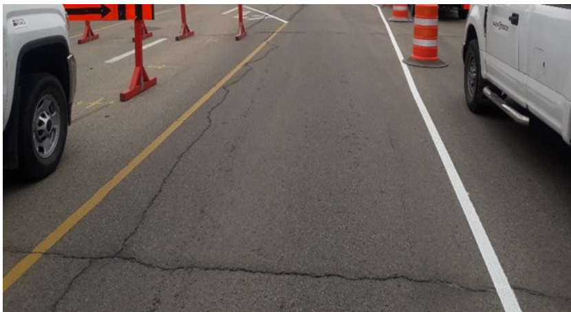
Figure 5: Installation of 3M Stamark Wet Reflective Removable Tape (Series 710)
