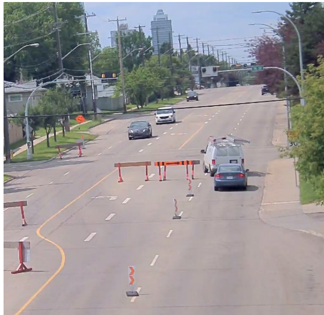
Figure 23: Left turn conflict at Site #1
