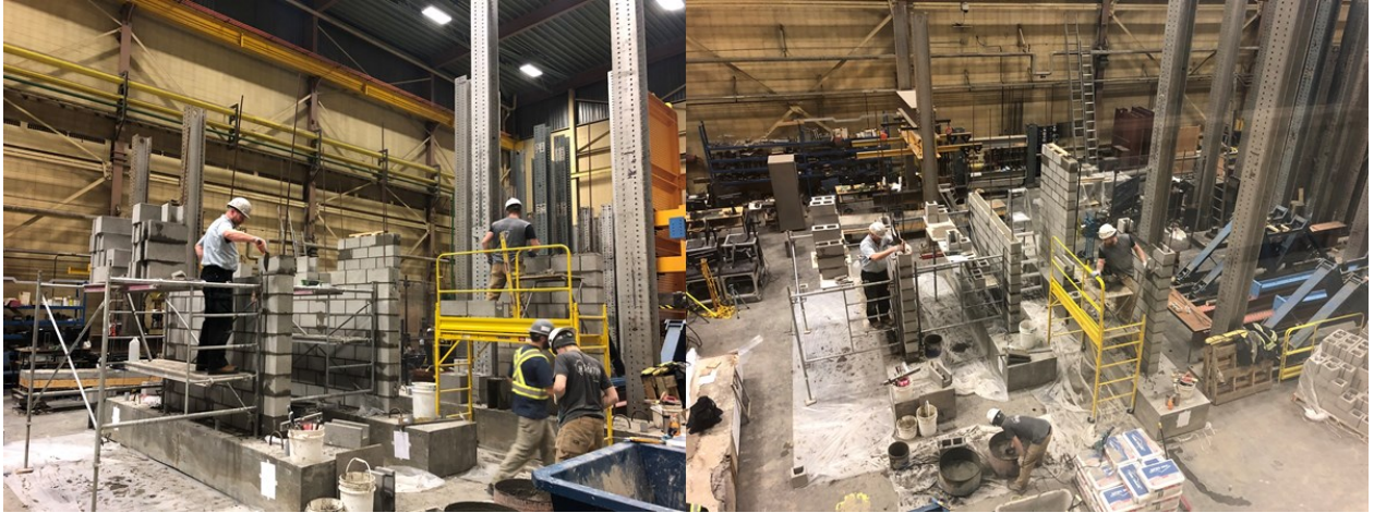
Figure A.12 Tested walls during construction
